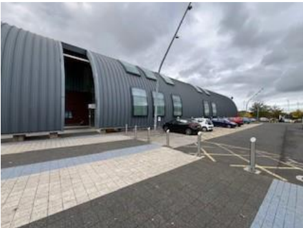
Disabled Parking 11 spaces to the front of the building in Parkland Gateway car park, NN17 1QG. 15 spaces to the side of the building in Victoria Car Park, NN17 1QE.
