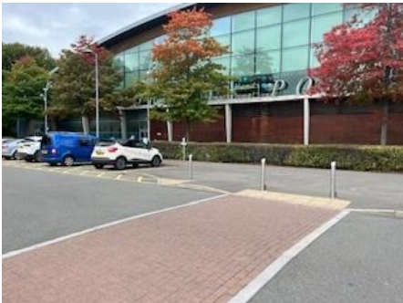
Drop kerb and one level access to facility.
